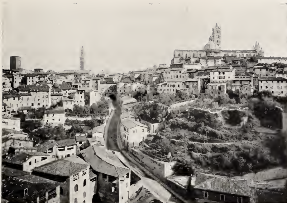
Illus. 284.—Siena. View showing general harmony of building materials used.
